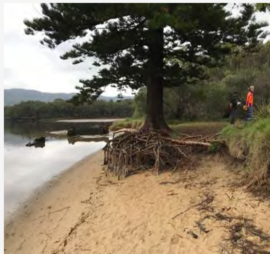
Coastal erosion (undermining of Norfolk Island pine)
